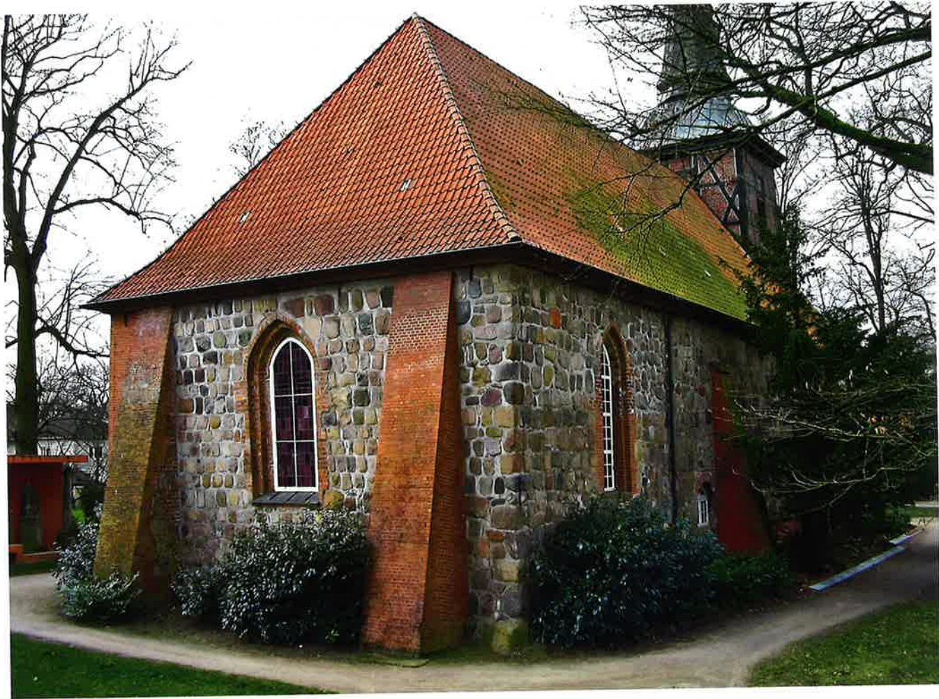
Fig. 2 The church at Bergsted in Stormarn retains essentially its original 12th century structure, with minor alterations (roof form, Late Gothic windows in brick mountings, an 18th century tower and west front, modern supporting pillars). According to a 13th century source it was dedicated to the Virgin Mary and St Wilhad, the patron saint of the cathedral church at Hamborg and the founder bishop of the diocese of Bremen respectively. The Virgin Mary came to be regarded as advocata et adiutrix of Holsten as a whole, as she was of other Baltic frontier zones like Prussia and Livonia.
